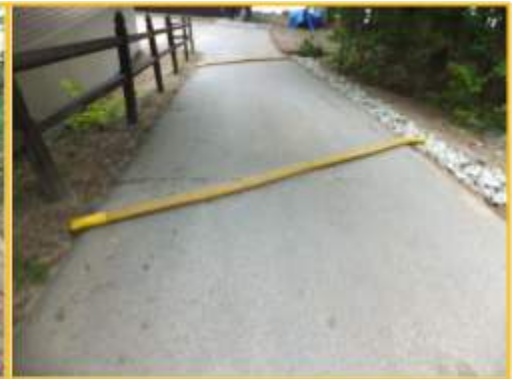
Firehose Diverter - In paved driveways, burying rubber and wood are not an option. Old firehose, or other durable material, can be filled with sand or stone and placed on an angle to divert stormwater. These have the added benefit of being movable.
