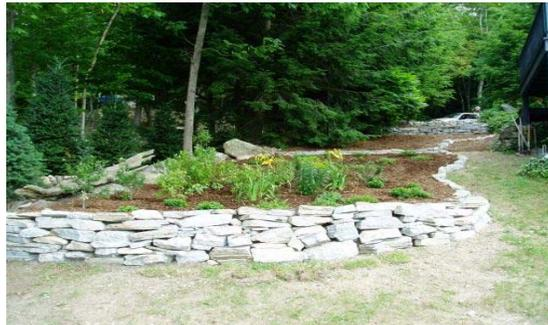
This beautiful and effective rain garden slows, catches and filters storm water runoff, correcting erosion patterns that formerly allowed the sediment to run into the lake.
